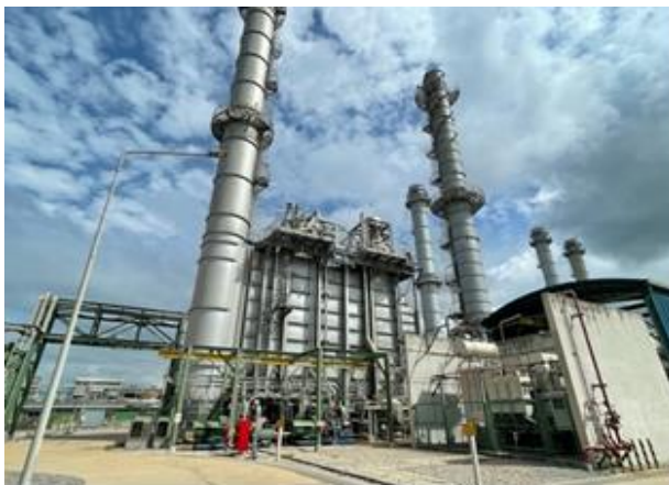
Heat Recovery Steam Generator (มี 6 Unit)
